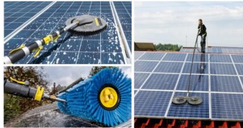
Fig. 4. Manual surface cleaning of solar PV modules
