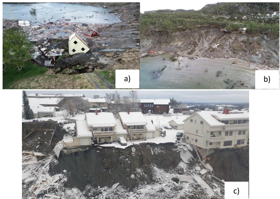
Fig. 4. Fast clay landslides: a - in Norway; b - in Kroknes near Alta; c - in Gerdrum (2020) [9]
